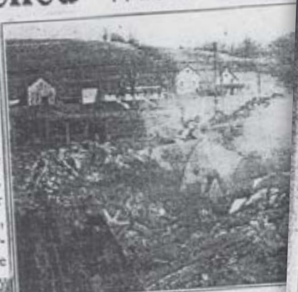
SHOWING PILES OF RUINED
