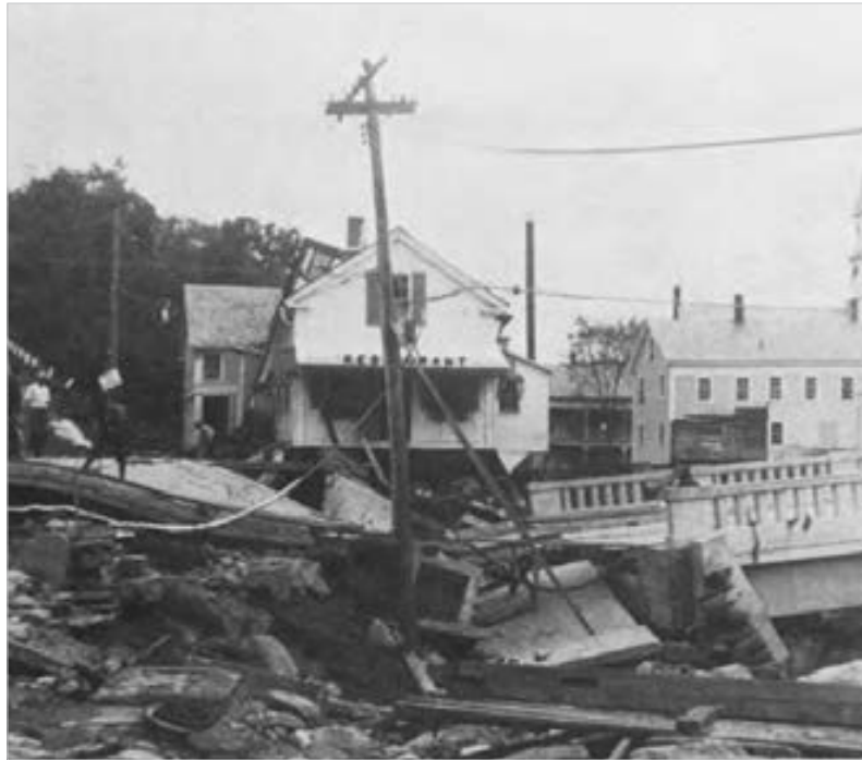
Above: The effects of the 1927 flood on West Main Street (left), and along the river's edge on South Main Street (right).
