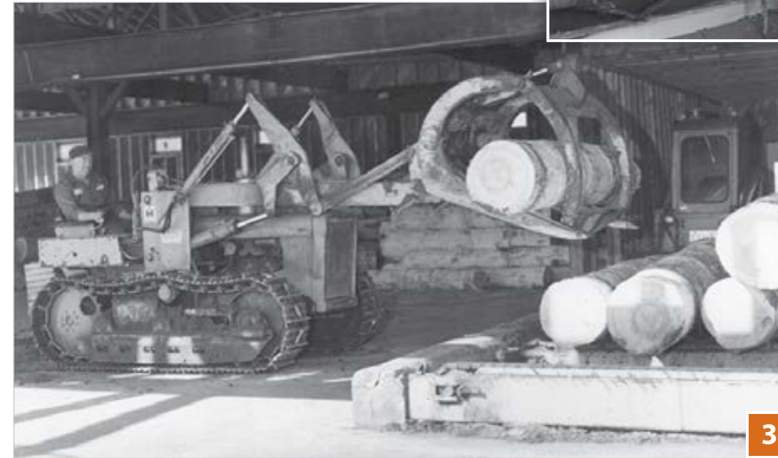
Logs started the production process in the newly-made log room (1) by being placed on the first live deck. The debarker stripped away the bark (2). Davis loaded debarked logs onto the second live deck (3) which sent them inside the factory.
