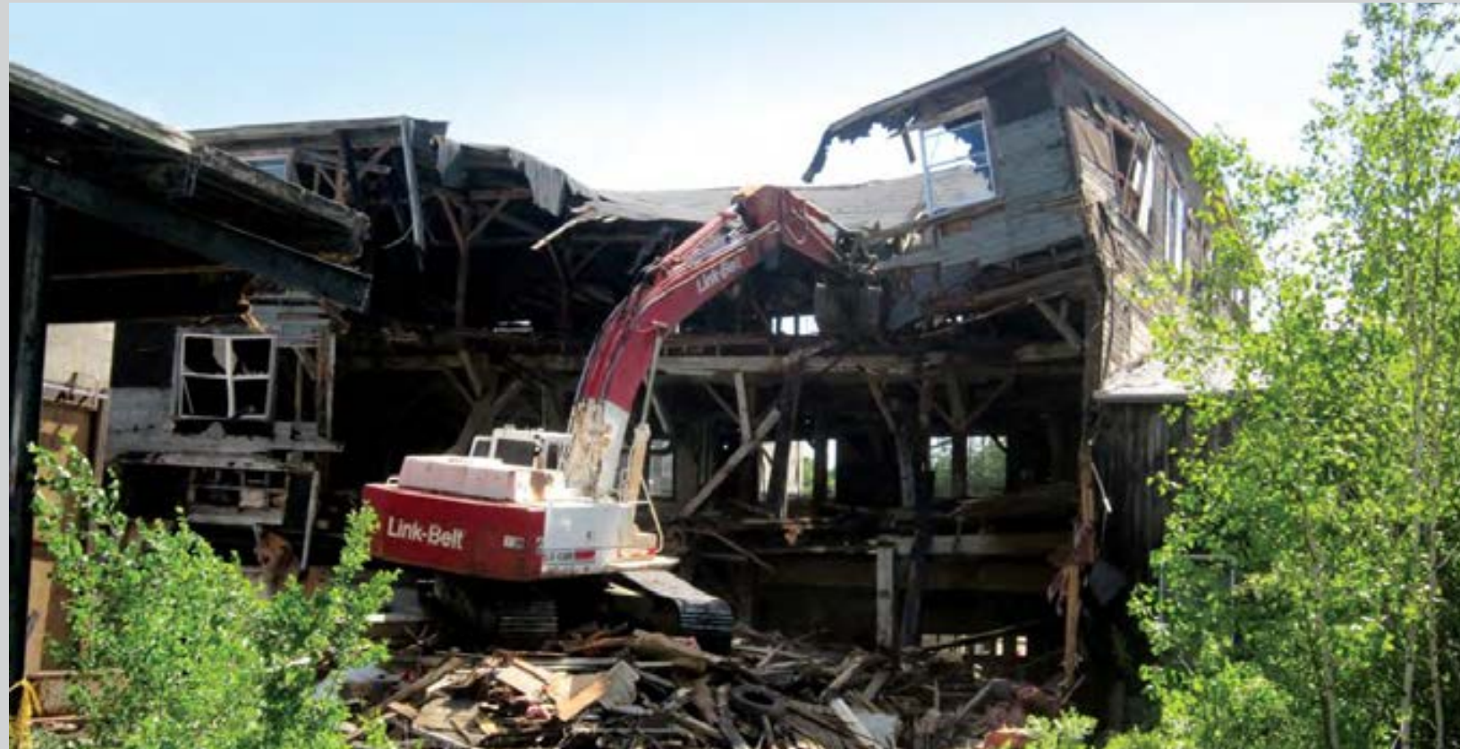
The three-story block began to visibly buckle in May 2011. It threatened the garage next to it and was condemned. An emergency demolition (below) took place in June 2011. The photo sequence shows the block's collapse as it is gutted from the opposite side by an excavator.
