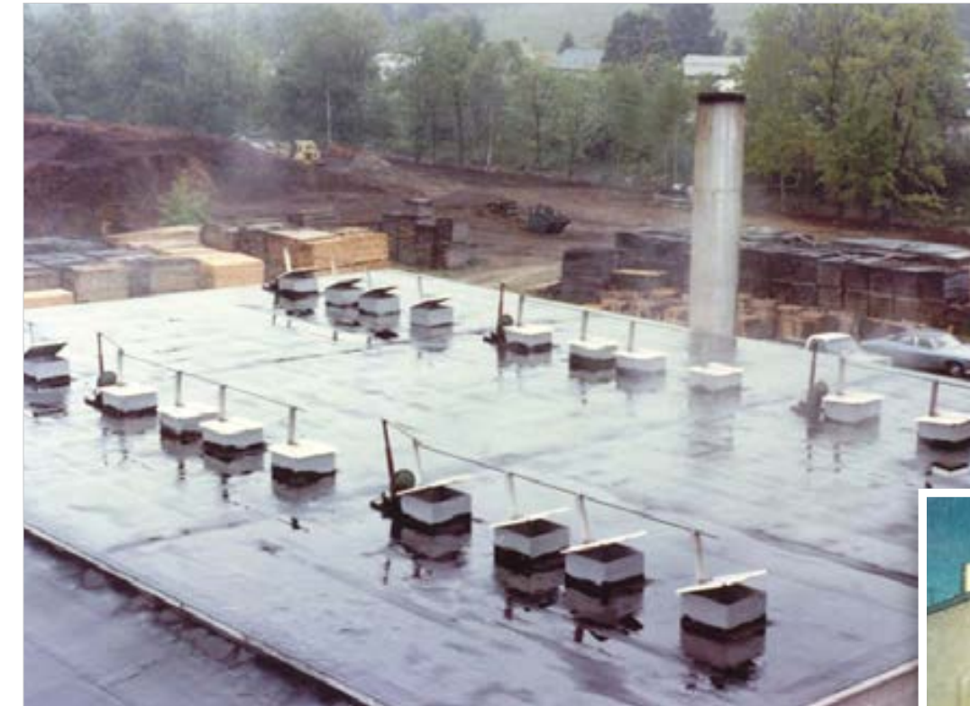
Left: The kiln roof vents and heat exchanger tower vent. Note the piles of finished product in the background and the end of a large bark mulch pile. Below: The kilns under construction.
