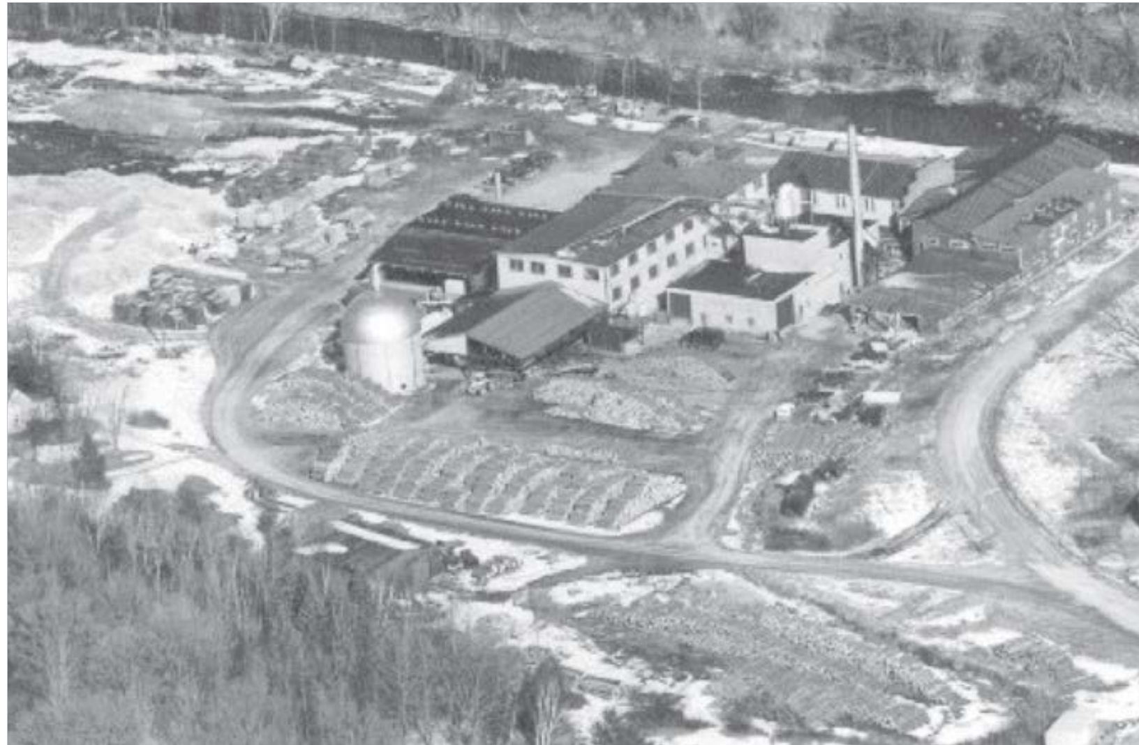
This aerial view was taken after the silo and boiler room complexes were built, but before the second sawroom was built (far right, just to the right of the smokestack). The foreground illustrates a recurring theme for 45 Mill Street – huge piles of logs. The factory started out using hardwood in the early 1900's and switched to softwood by the late 1900's. The rail spur changed to an entry road (center) while a new road (far right) was added and nicknamed Plywood Street during the New England Box Company days. Note the series of pipes along the roofs of the main block and boiler room that collected sawdust for the huge boiler.
