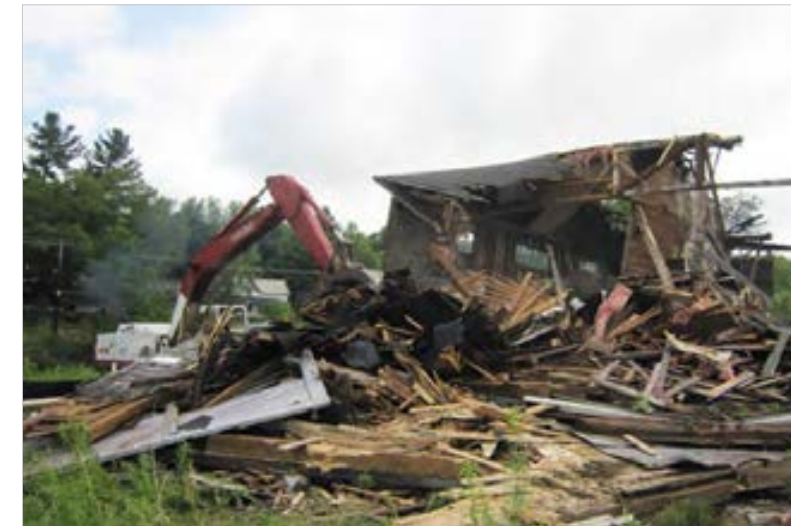
Above: Demolition resumed in July 2011 and site clean-up continued throughout that summer. First, the kilns were torn down (upper left), then the circa 1925 building (upper right), and finally the 1916 offices section (lower left). After the buildings hit the ground, they were plowed into a debris pile (lower right) to begin the material recovery and recycling process.
