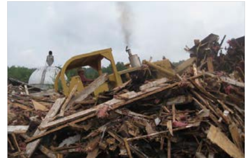
Above: Demolition resumed in July 2011 and site clean-up continued throughout that summer. First, the kilns were torn down (upper left), then the circa 1925 building (upper right), and finally the 1916 offices section (lower left). After the buildings hit the ground, they were plowed into a debris pile (lower right) to begin the material recovery and recycling process.
