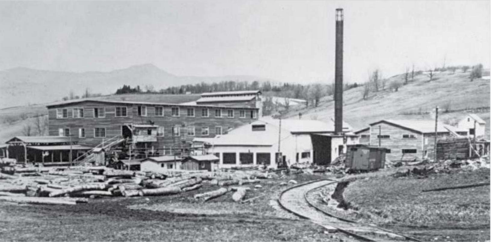
Below: Logs are piled in the yard randomly before processing; later, a log pond was built there. The two-story building at the far right housed many functions over the years and collapsed in the spring of 2008.
