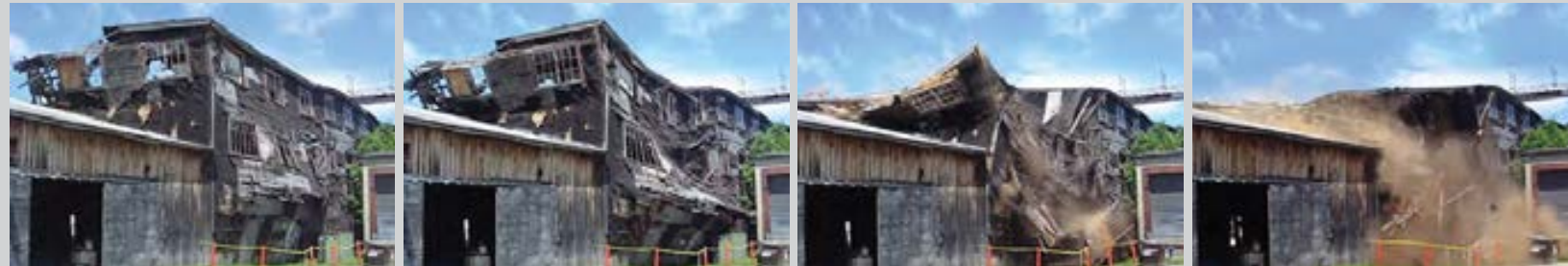
The three-story block began to visibly buckle in May 2011. It threatened the garage next to it and was condemned. An emergency demolition (below) took place in June 2011. The photo sequence shows the block's collapse as it is gutted from the opposite side by an excavator.
