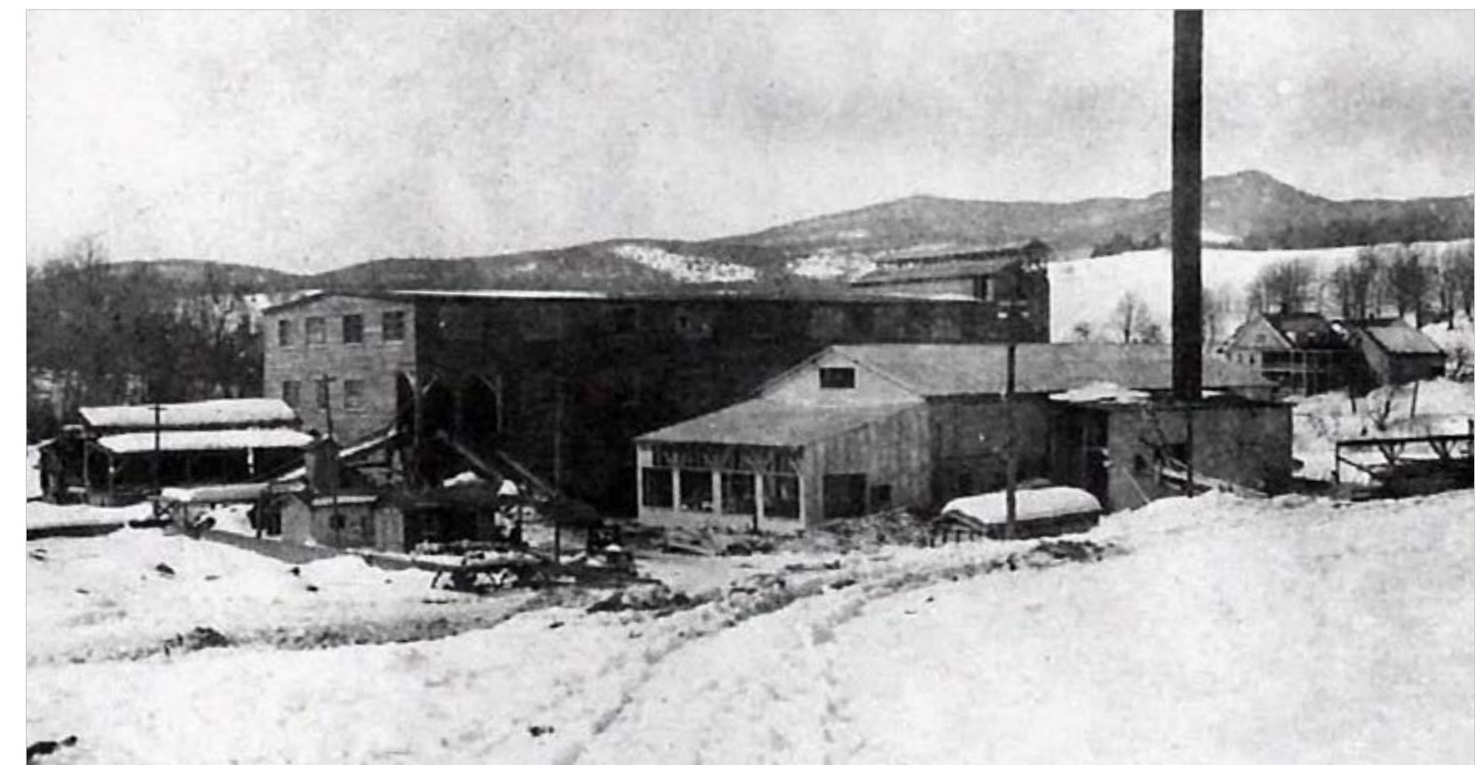
Below: The second mill. This photo shows the conveyors in and out of the three-story building and the new, smaller woodworking building (right).
